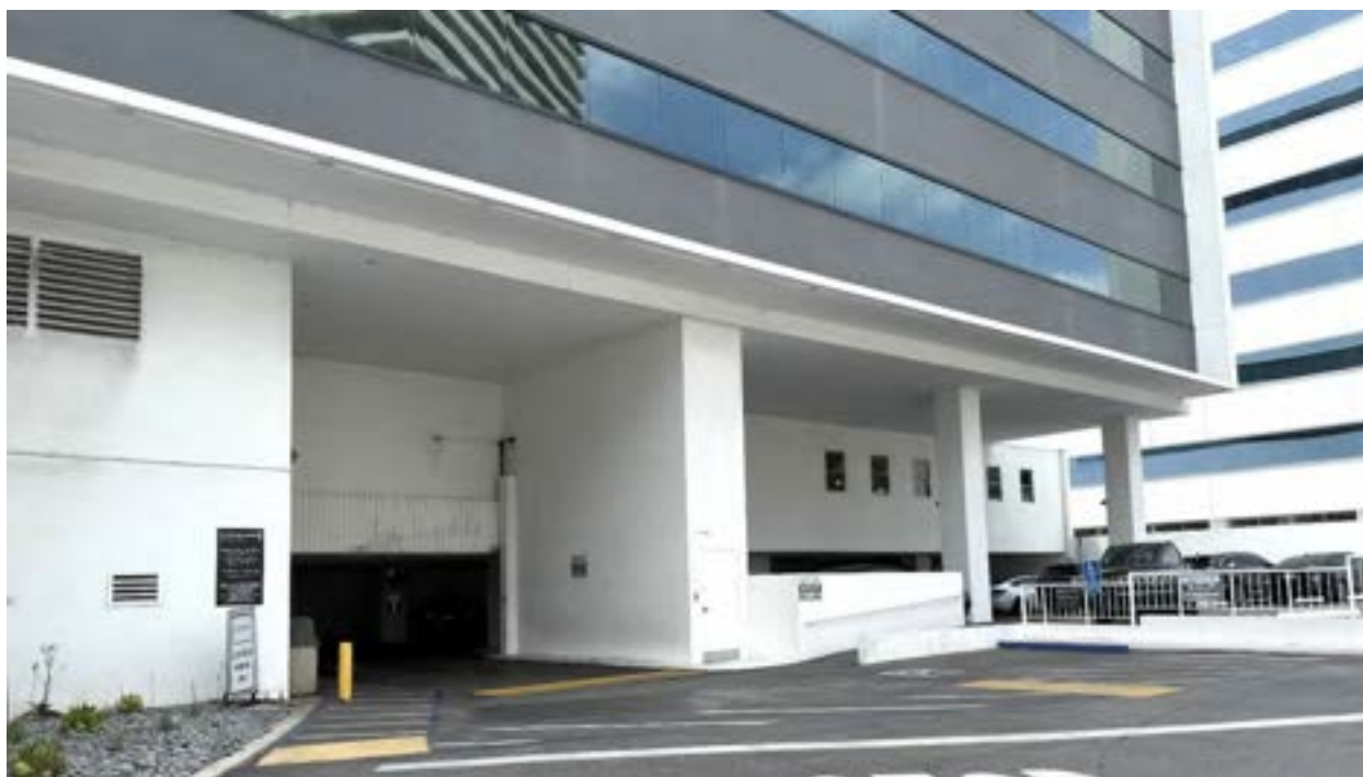
Figure 9: North (rear) elevation of commercial building, view looking south. GPA, May 2025.
