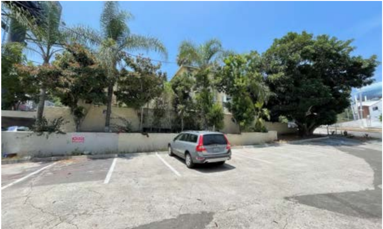
South façade and parking lot, view northeast
