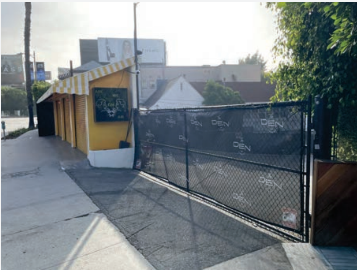
Photo 3. Subject property's primary (north) and west side facades, view northeast.
