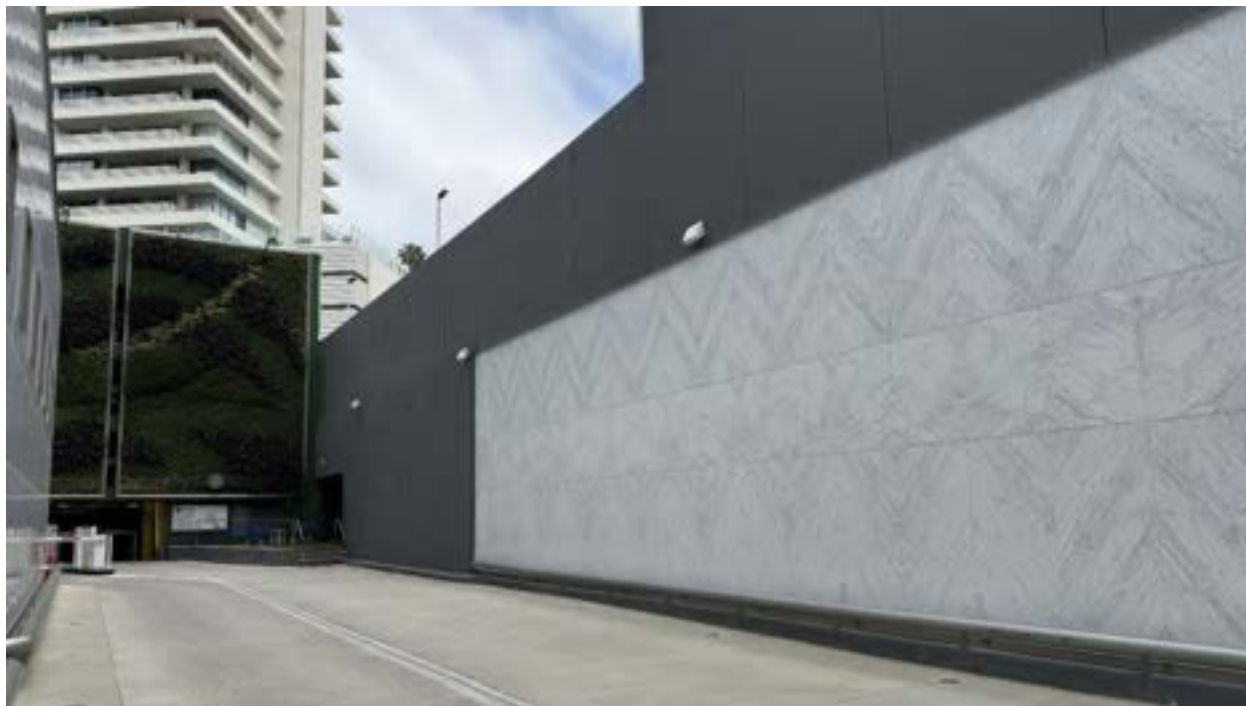
Figure 12: West (side) elevation of commercial building, view looking north. GPA, May 2025.
