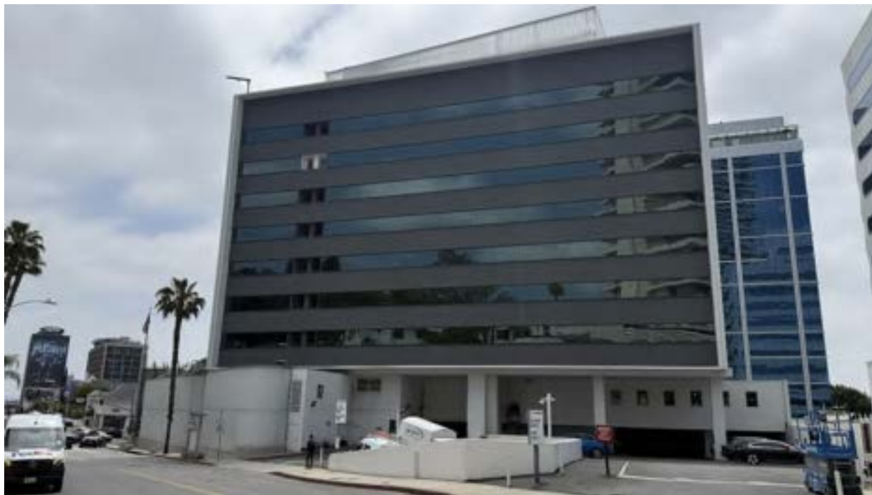
Figure 8: North (rear) elevation of commercial building, view looking southeast. GPA, May 2025.
