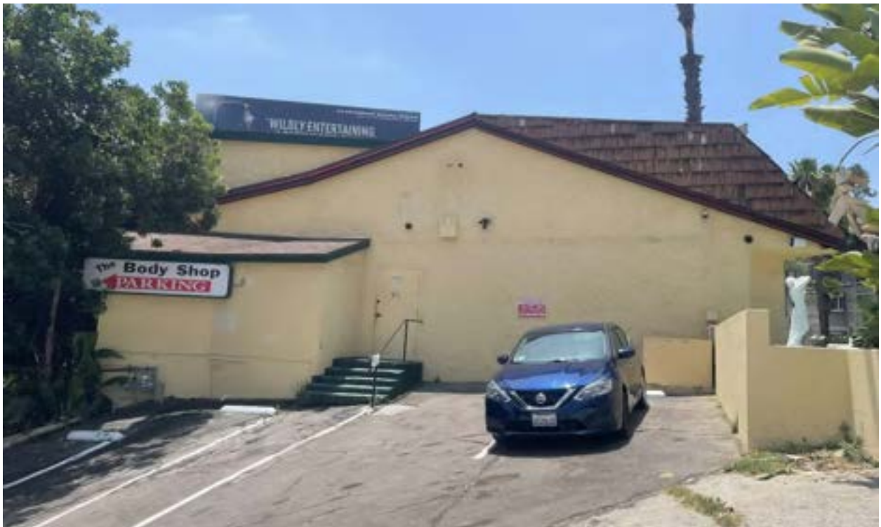
East façade, view west from North Harper Avenue
