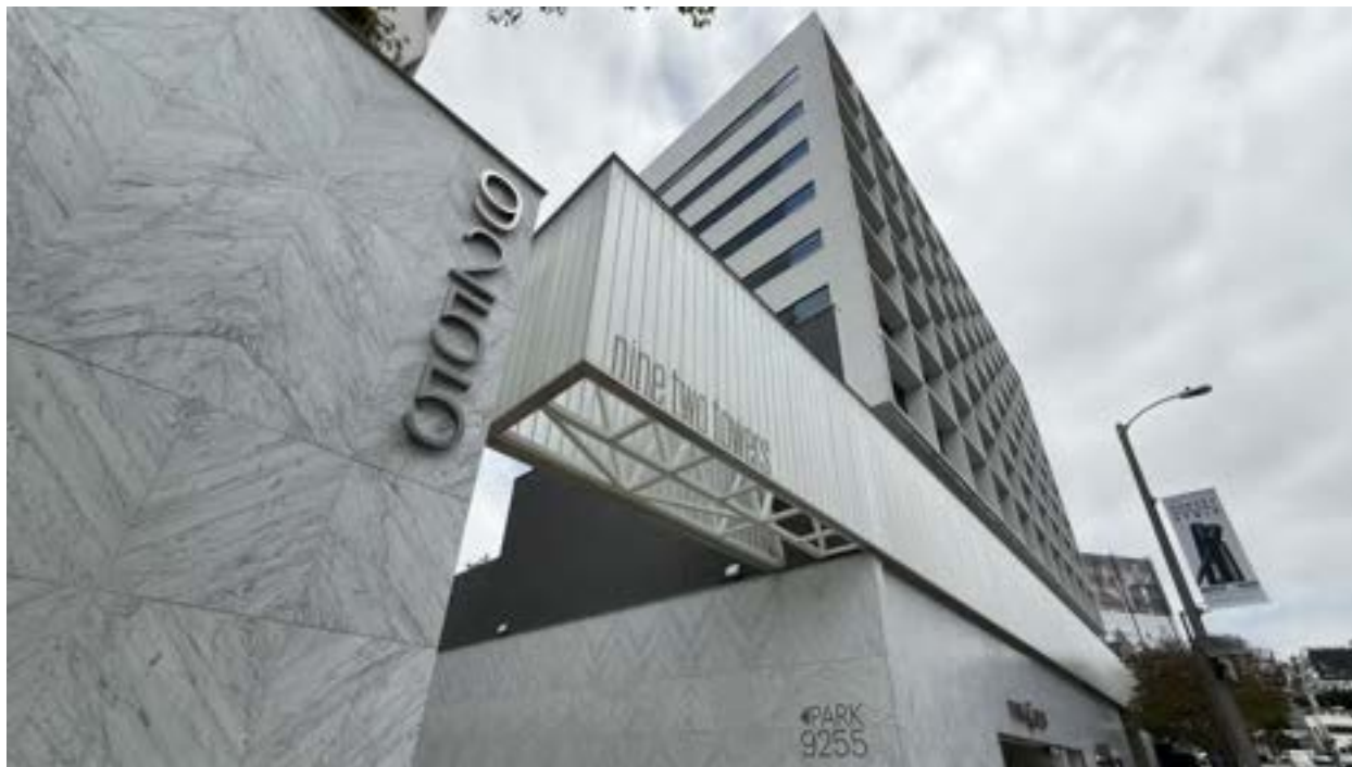
Figure 10: West (side, at left) and south (primary, at right) elevation of commercial building, view looking northeast. GPA, May 2025.
