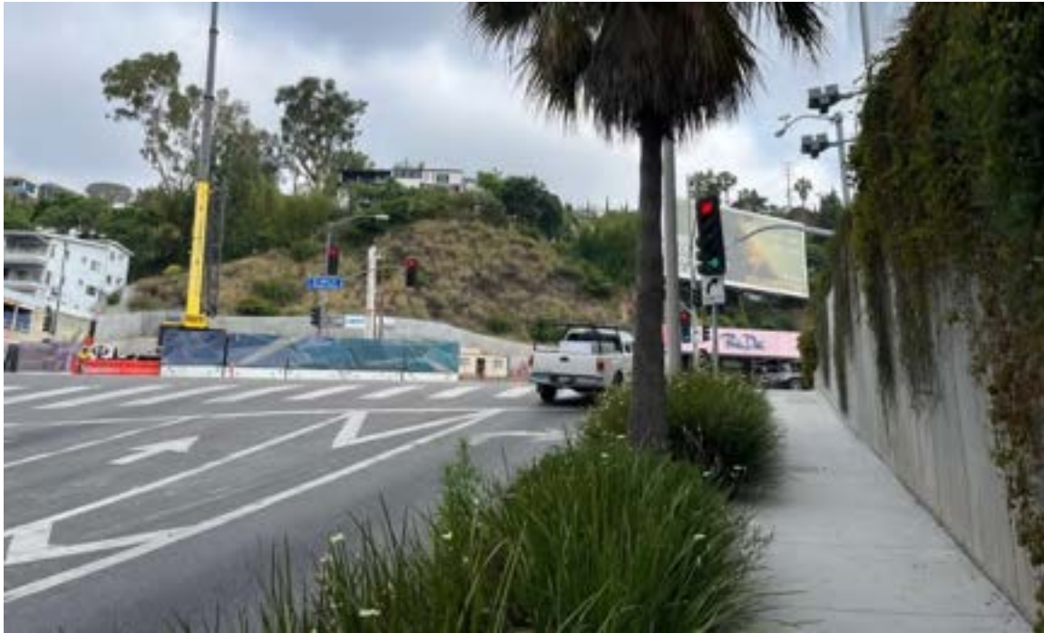
Figure 3 Project Site at Sunset and La Cienega Showing Right Turn Overlap Phase
