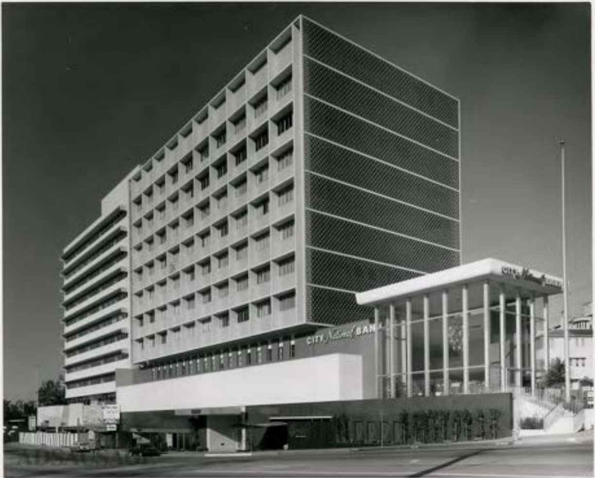
Figure 13: Subject building, c. 1961, view looking northwest. Historic photo courtesy of Adsasusage Los Angeles Photo Archive, www.adsasusage.com
