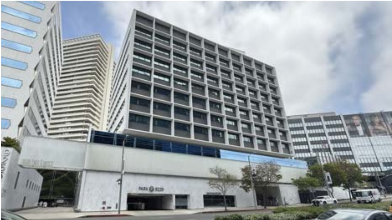
Figure 2: South (primary) elevation of commercial building, view looking north. GPA, May 2025.
