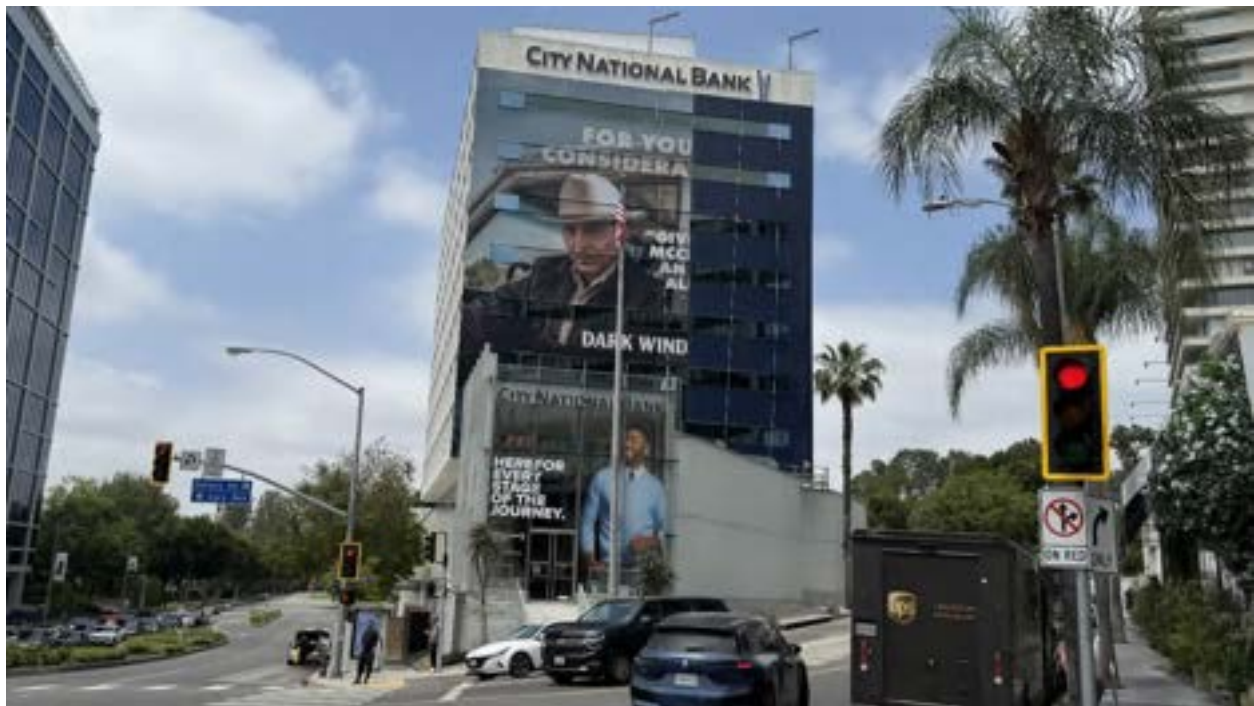
Figure 5: East (side) elevation of commercial building, view looking southwest. GPA, May 2025.
