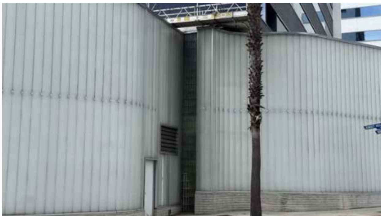
Figure 7: North (rear) elevation of commercial building, view looking south. GPA, May 2025.
