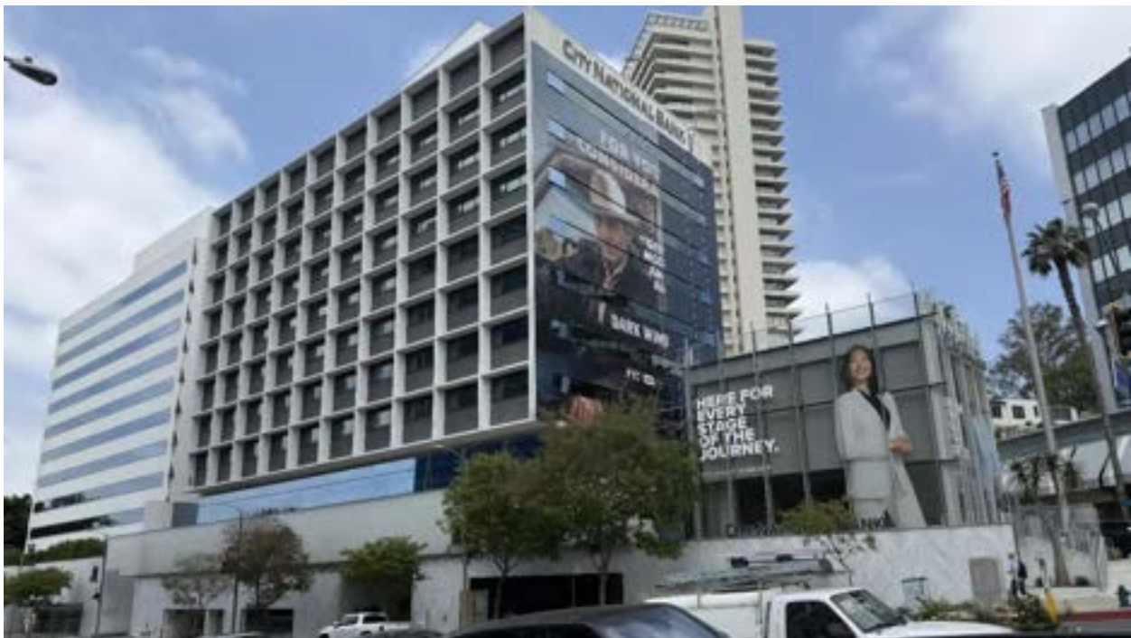
Figure 3: South (primary, at left) and east (side, at right) elevations of commercial building, view looking northwest. GPA, May 2025.
