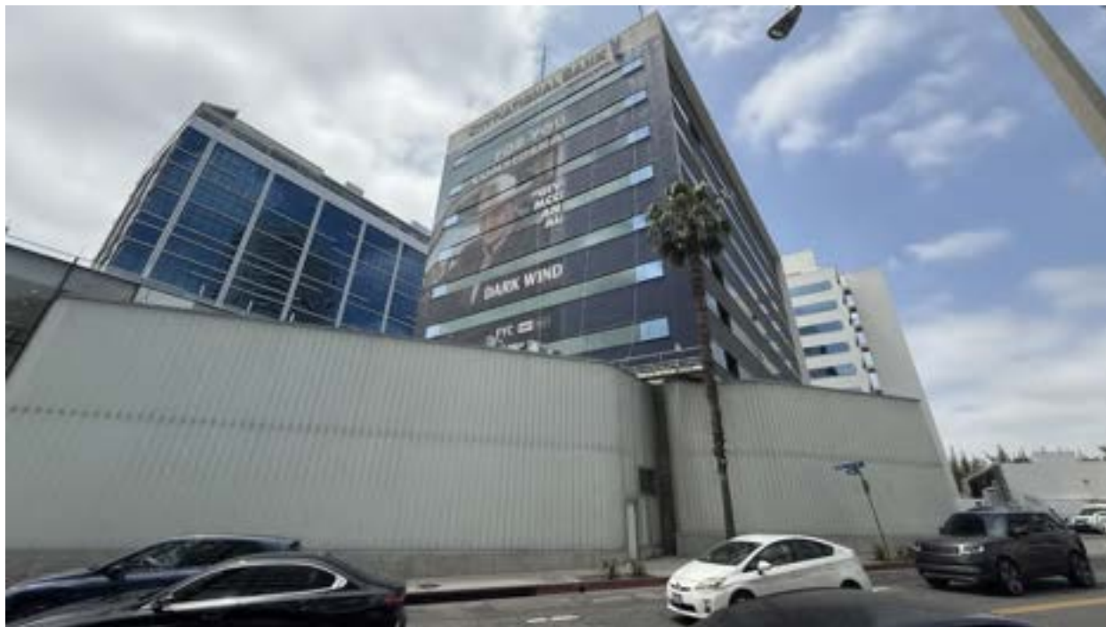
Figure 6: East (side, at left) and north (rear, at right) elevations of commercial building, view looking southwest. GPA, May 2025.
