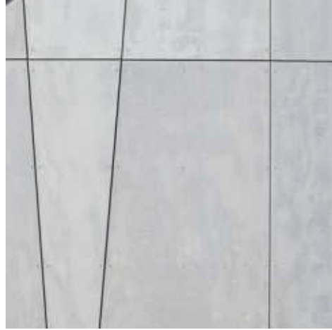
01. PRECAST CONCRETE PANELS
