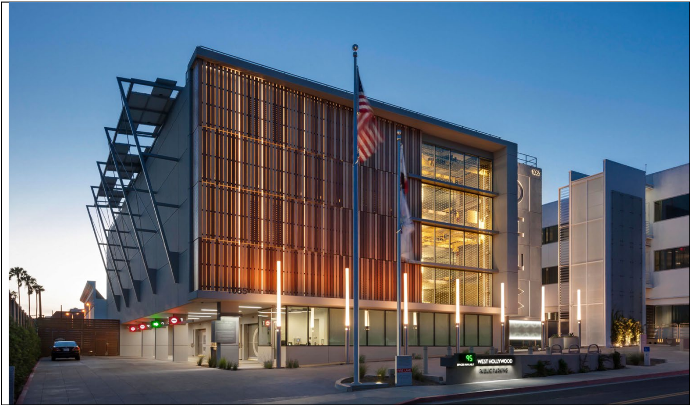
Exterior approach view to WEHO fully automated parking garage.
