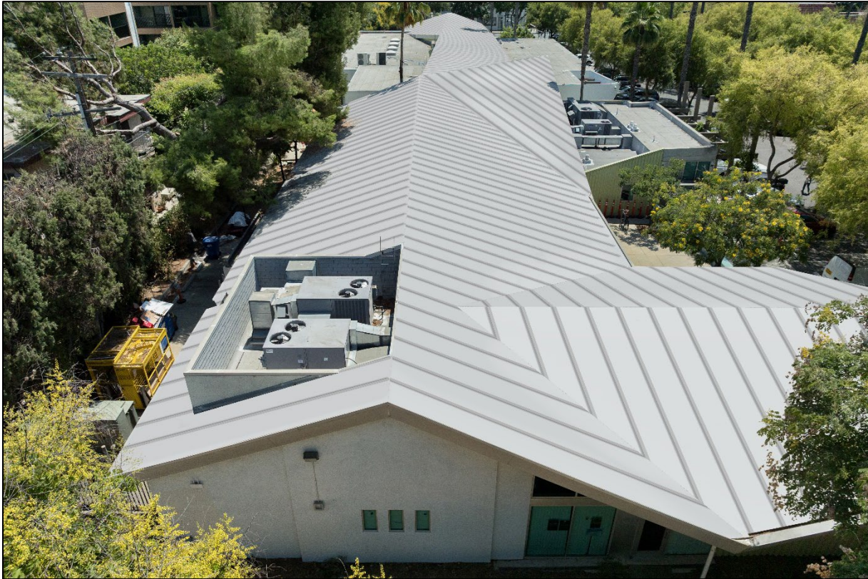
North Elevation Looking South
