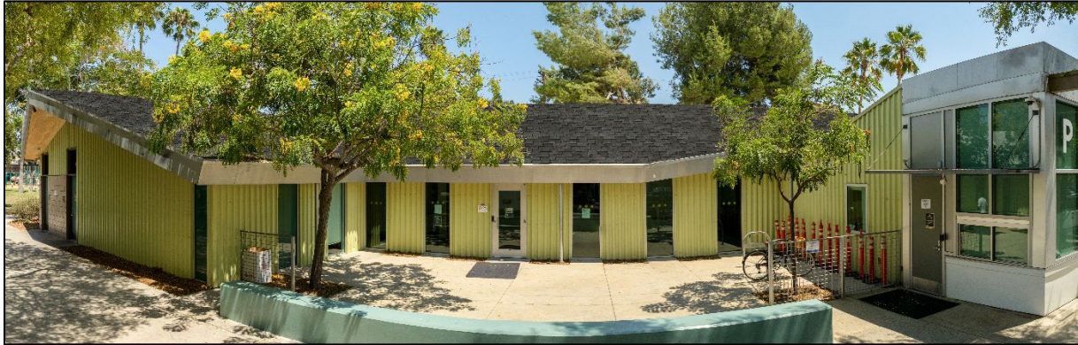
North Courtyard Looking East
