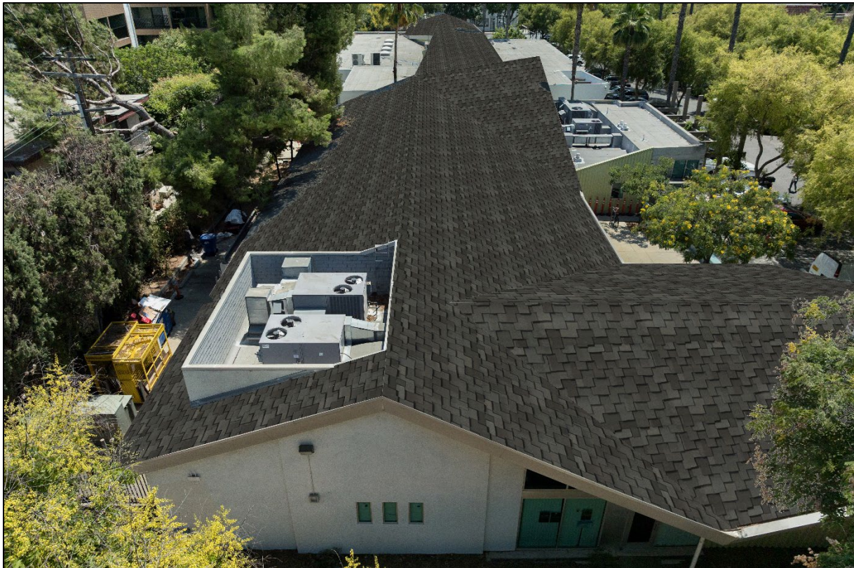
North Elevation Looking South
