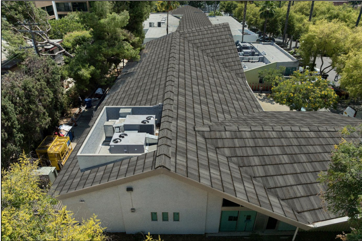
North Elevation Looking South
