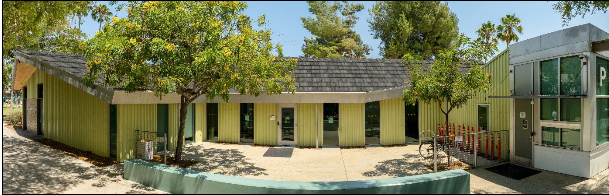
North Courtyard Looking East
