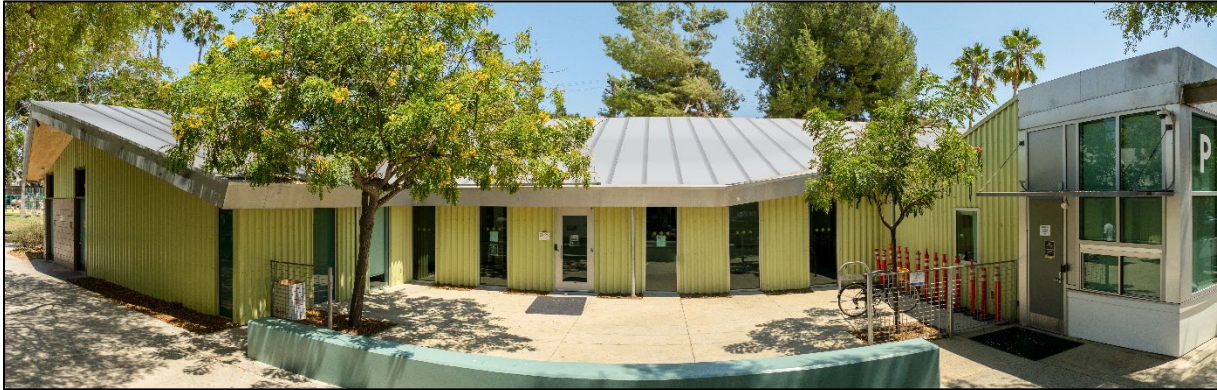
North Courtyard Looking East
