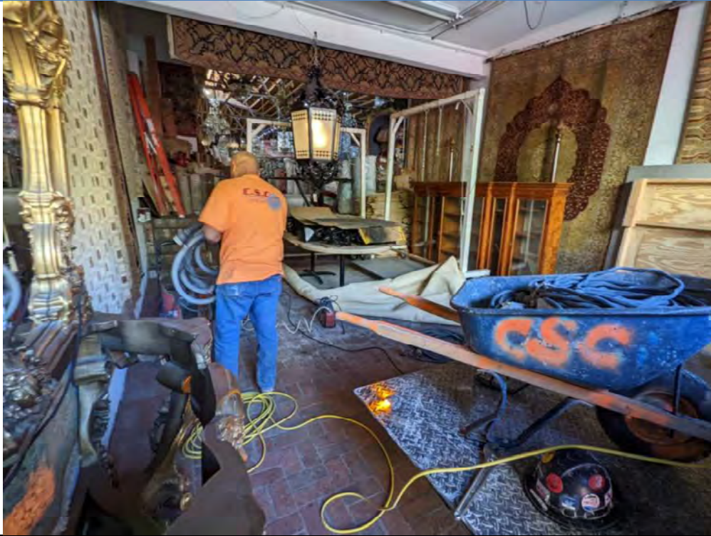
PHOTO 1: Cement coring at boring location B1 (3/11/22).
