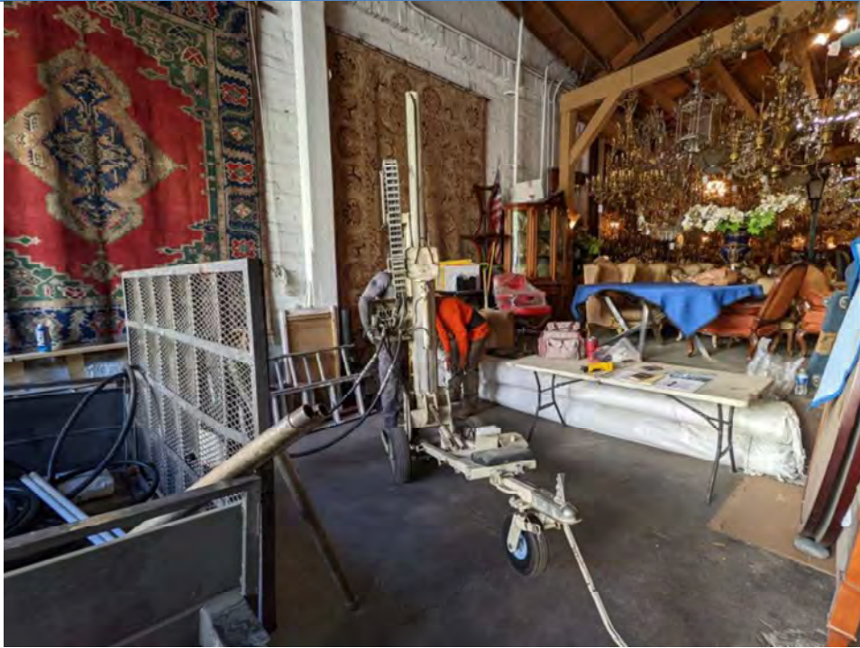
PHOTO 3: Drilling operations at boring location B3 (3/11/22).
