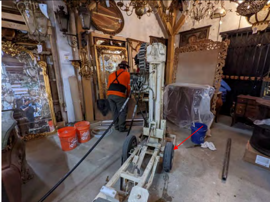
PHOTO 4: Drilling operations at boring location B4 (3/11/22).
