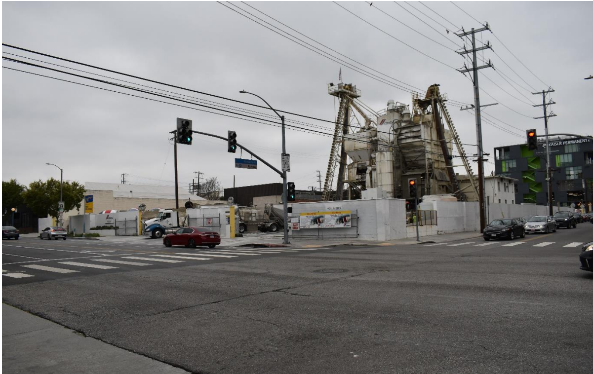
Figure 3 View of Project Site from North La Brea Avenue looking Northeast
