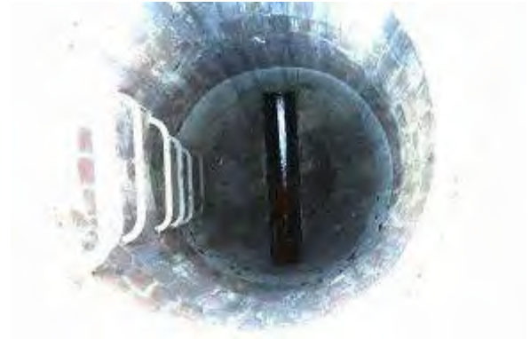
Manhole Before Install
