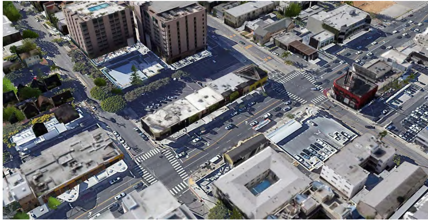
AERIAL VIEW SHOWING EXISTING SITE FROM THE NORTHWEST
