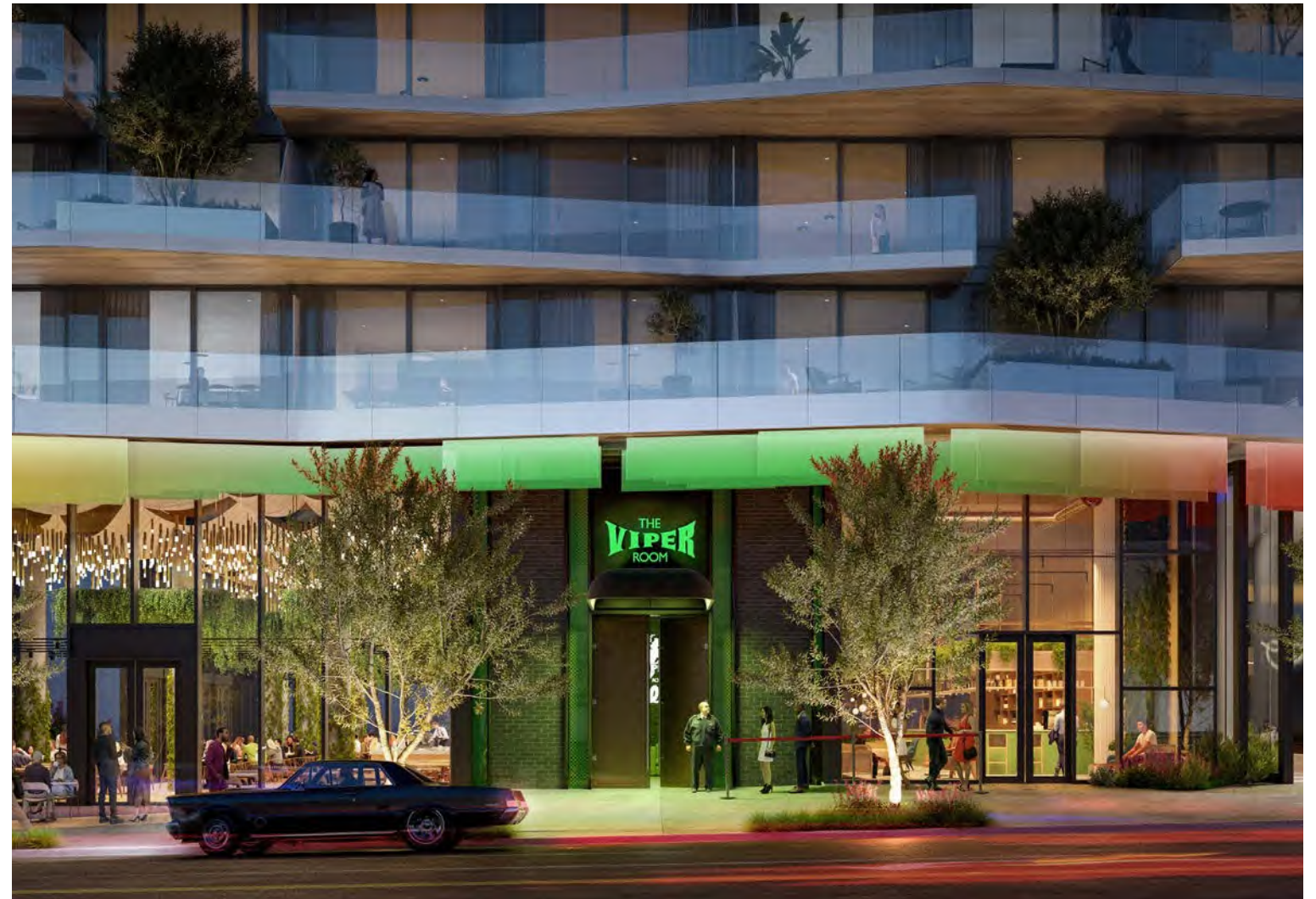
VIEW OF CANOPY LIGHTING FEATURE ALONG SUNSET IN FRONT OF VIPER ROOM
