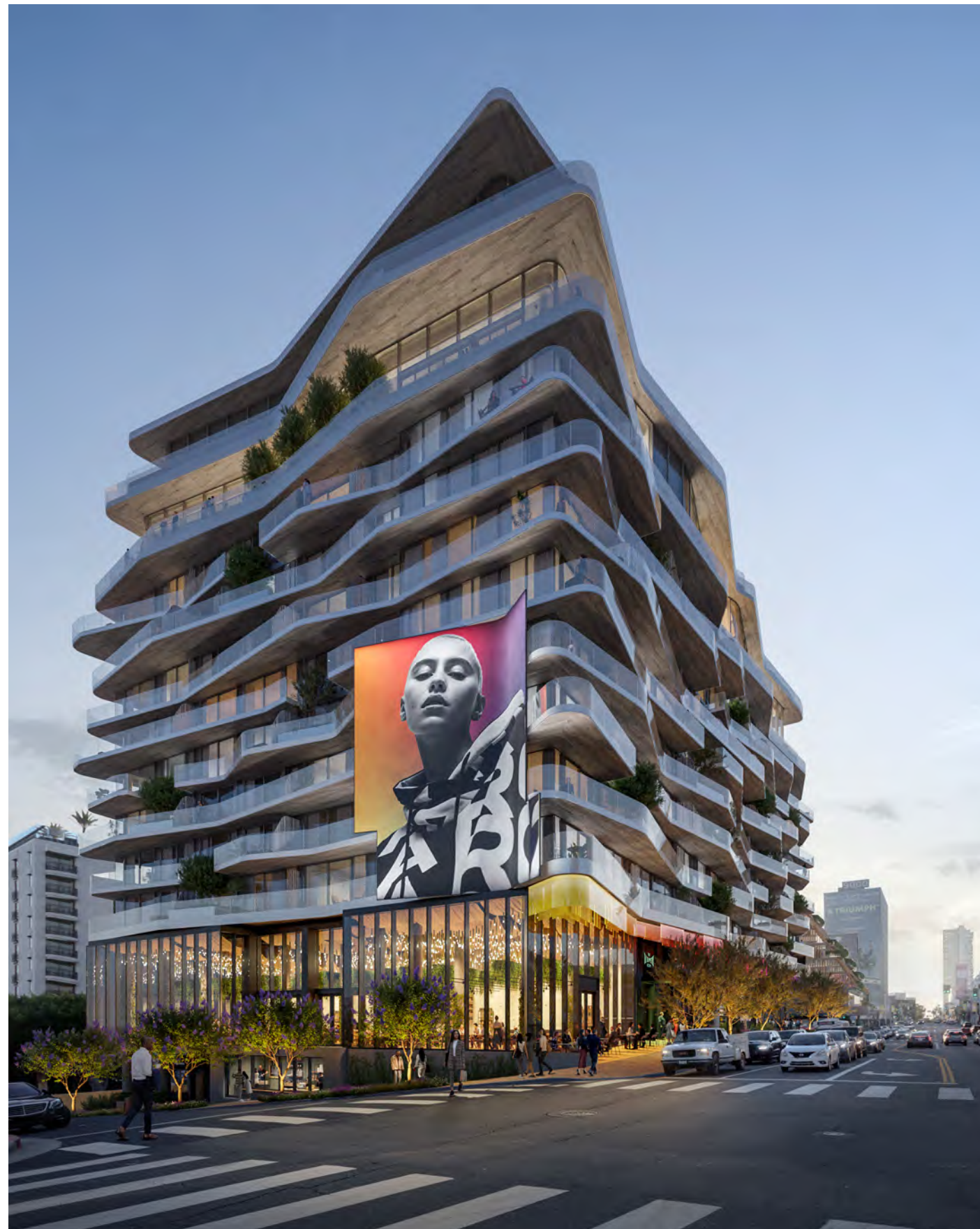
VIEW AT NORTHEAST CORNER OF BUILDING
