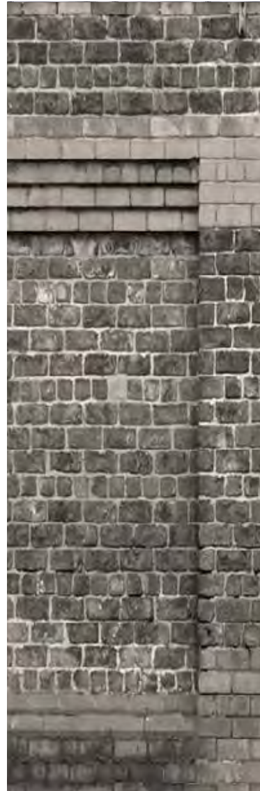
BLACK BRICK WALL
