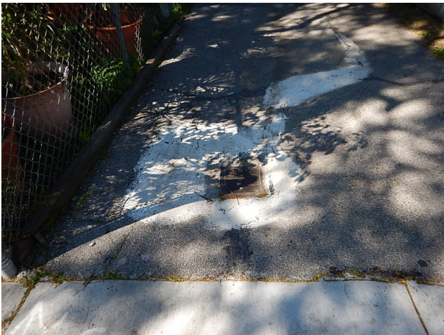
19. View of storm drain at subject property
