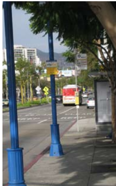
Improvements made to Santa Monica Boulevard have enhanced its role as a transit corridor.
