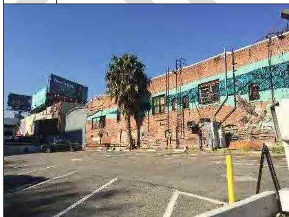
9. Parking area behind the eastern commercial buildings on the northern half of the Subject Property.
