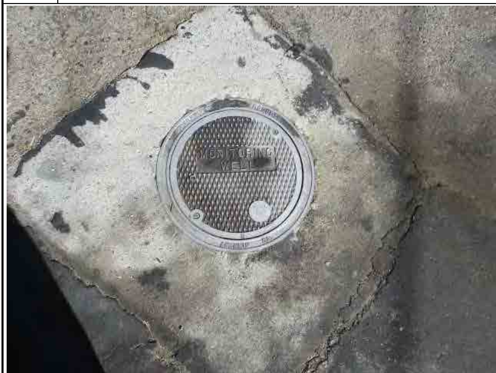
14. Typical groundwater monitoring well at the site.
