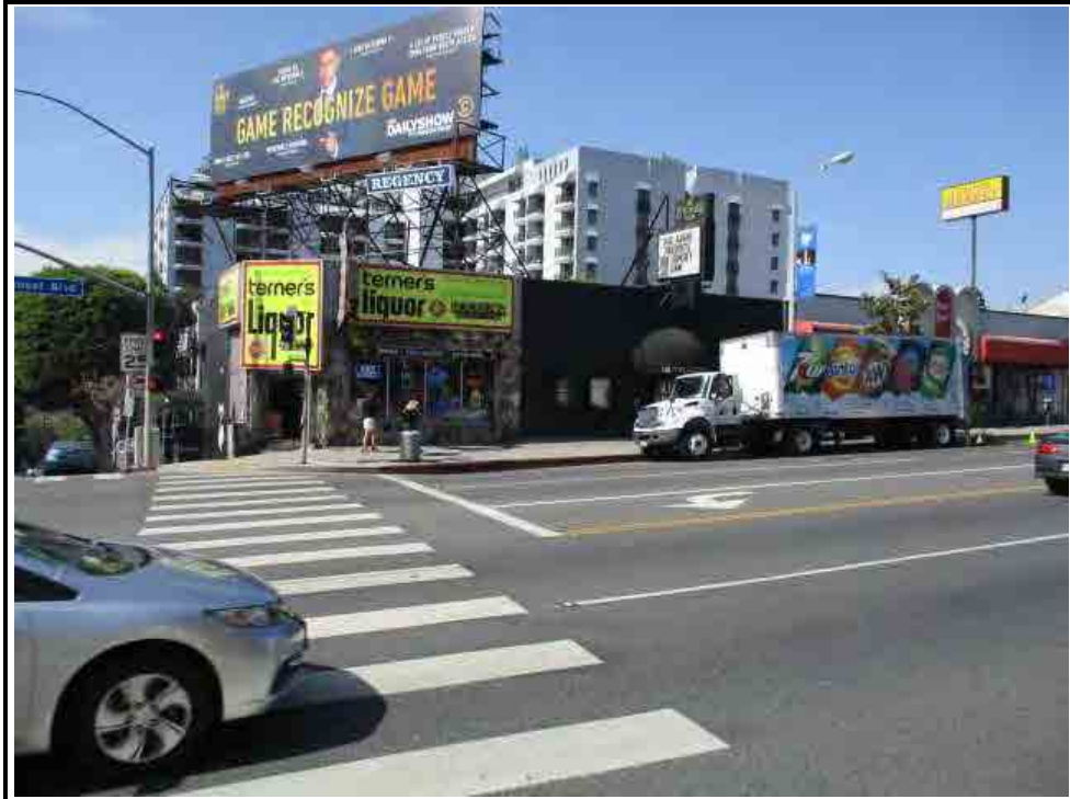
3. North façade of 8850-8860 W. Sunset Boulevard building.
