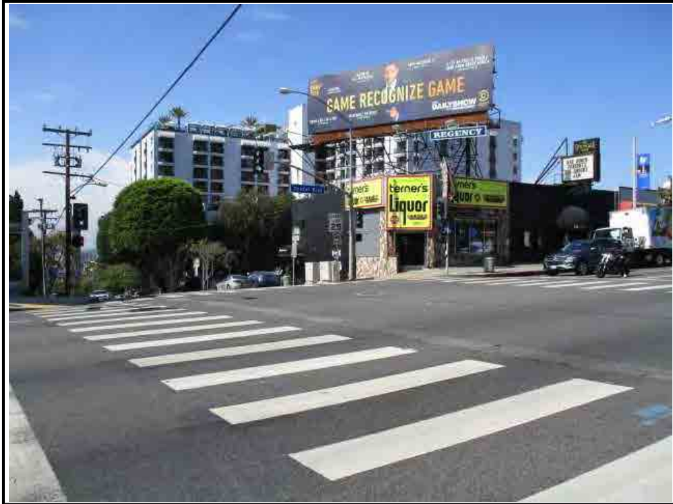
7. East façade of 8850-8860 W. Sunset Boulevard building.
