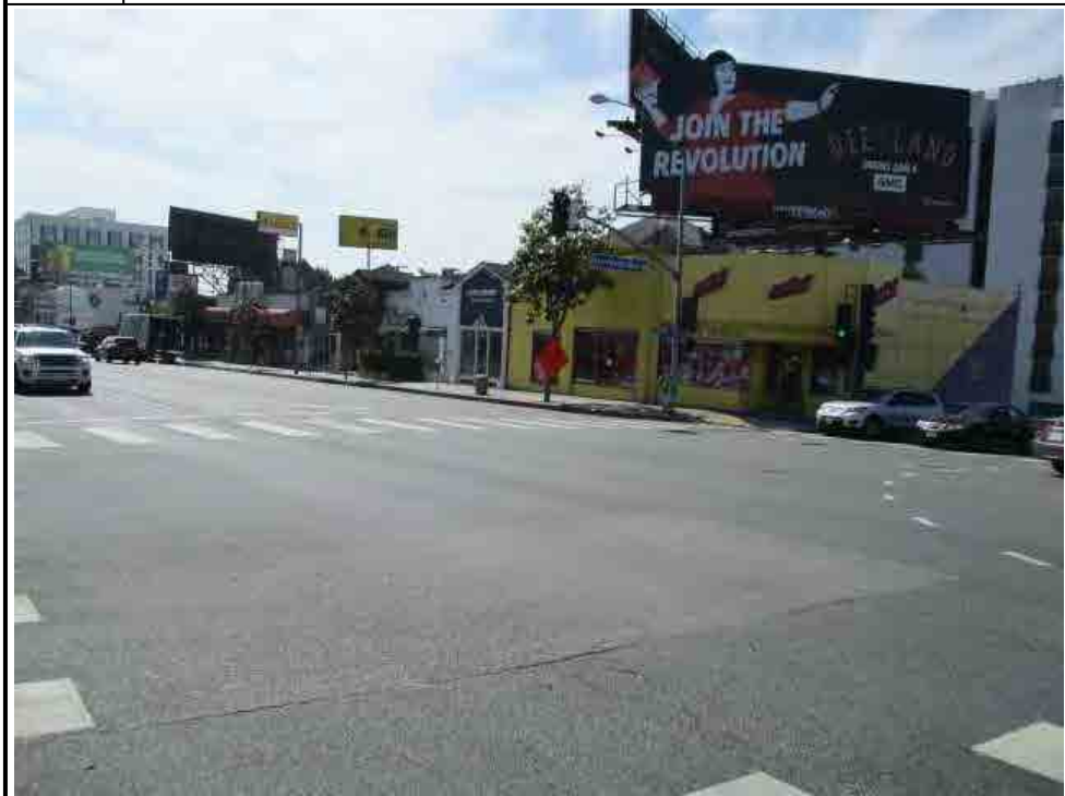
2. North facade of the building.
