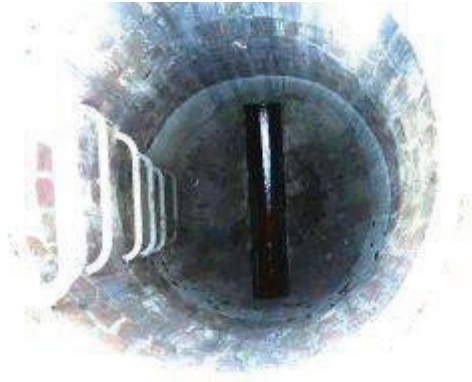
Manhole Before Install
