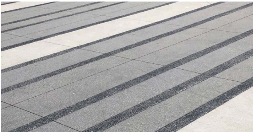
Paving - Integral color concrete and concrete pavers
