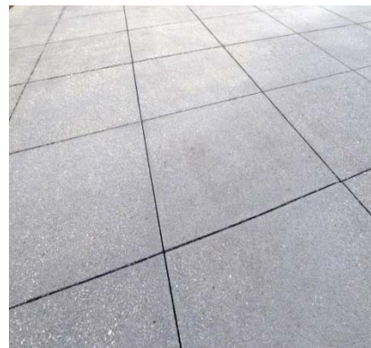
'Alternate' Decorative Concrete with a integral cool gray color & sandpaper finish
