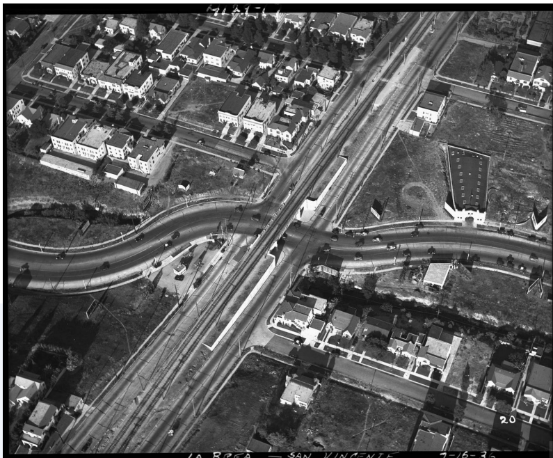
Though planning on Crenshaw North only kicked off in the 2000s, the communities it will run through (Crenshaw, Mid City, West Hollywood, and Hollywood) were built around historic Pacific Electric Streetcar lines like this one at San Vicente/ La Brea in 1936 (Metro Library).
