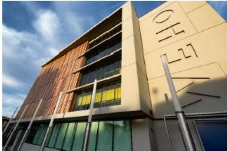
Automated Parking Garage. Photo Credit: Jon Viscott
