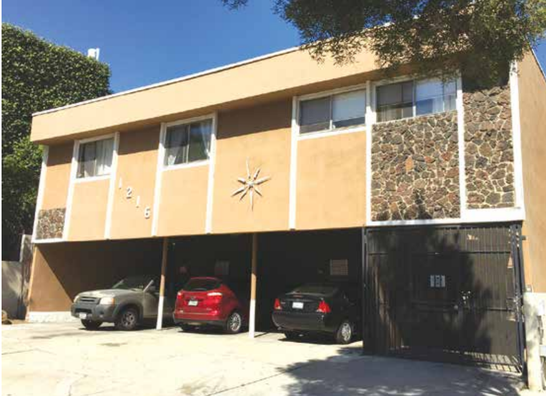
Apartments with parking under the first level along the street frontage
