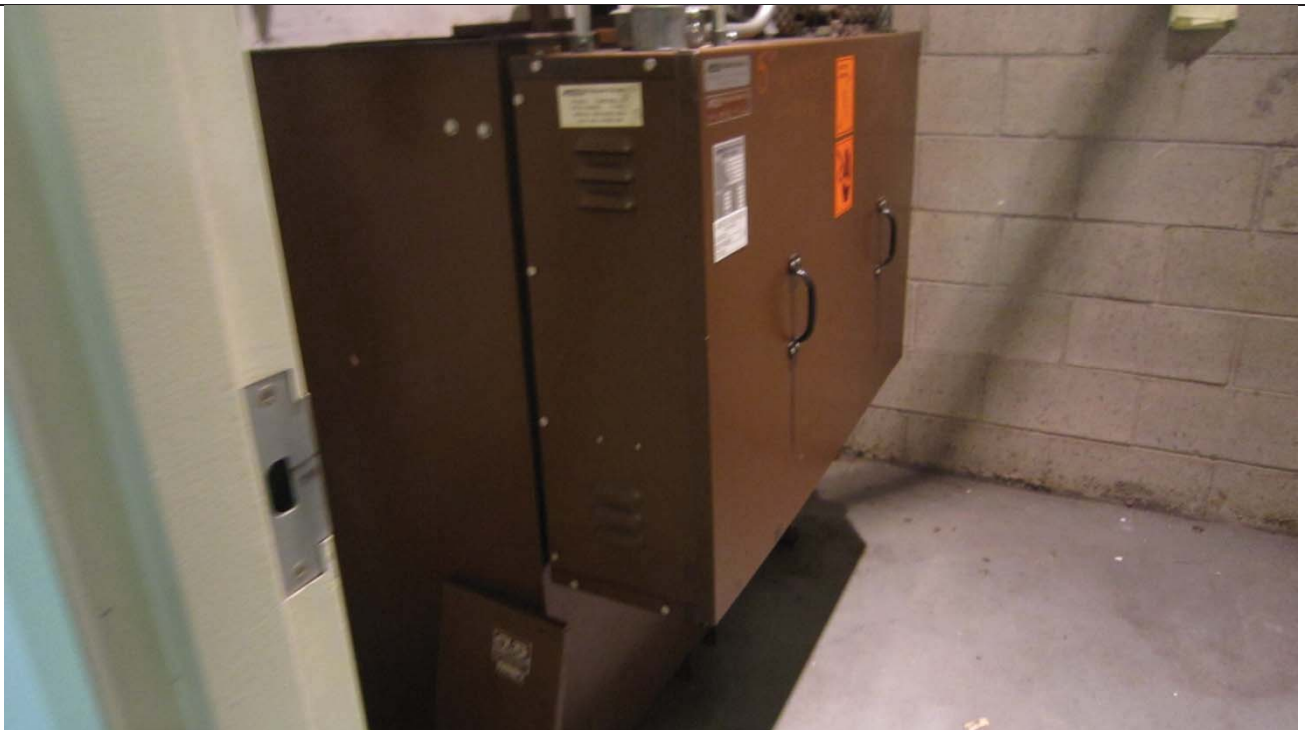
PHOTO 4: View of the elevator room on Level P1.
