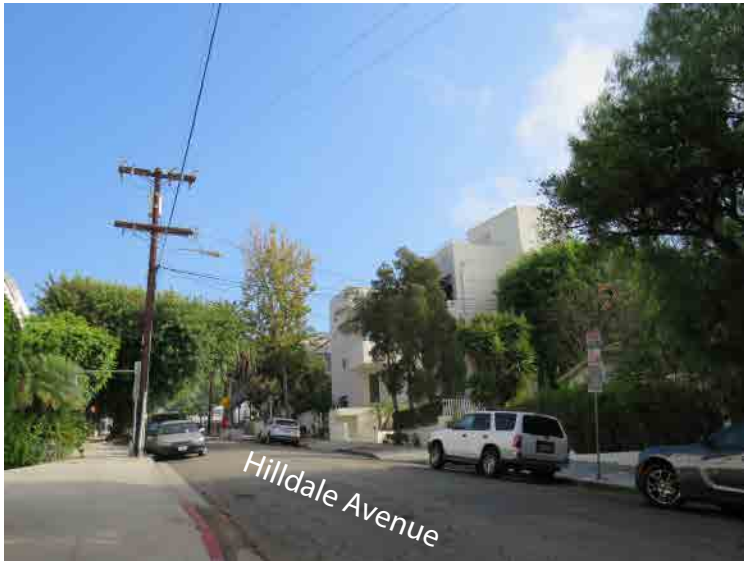
Multi-family residential uses on Hilldale Ave. immediately south of the Project Site.
