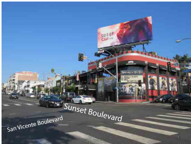
Commercial uses on the north side of Sunset Blvd. across from the Project Site looking northwest from Sunset Blvd. and San Vicente Blvd./Clark St.
