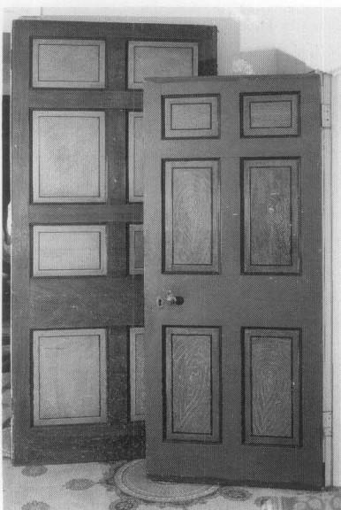
Figure 6. Historic doors may have graining patterns or clear finishes under one or several coats of plain paint, such as these restored 18th and early 19th century doors. Graining may appear even on more vernacular doors of the pre-1850 vintage. Photo: Jack E. Boucher for HABS.
