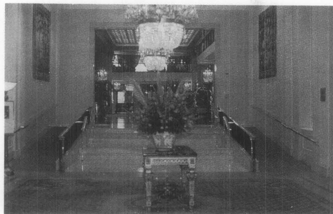
Figure 18. Symmetrical ramps at the Mayflower Hotel in Washington, D.C., provide access to the hotel's lower level. The design for the ramps respects the historic character of this landmark building. Photo: Thomas Jester.
