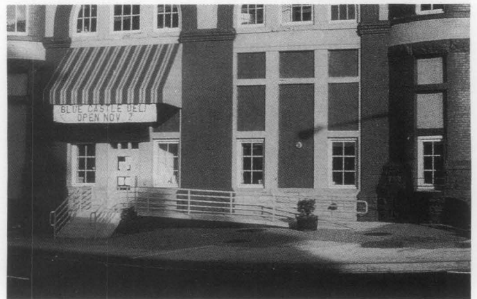
Figure 11. Simple, contemporary railings that extend beyond the ramp slope make this ramp compatible with the industrial character of this building. Photo: Thomas Jester.
