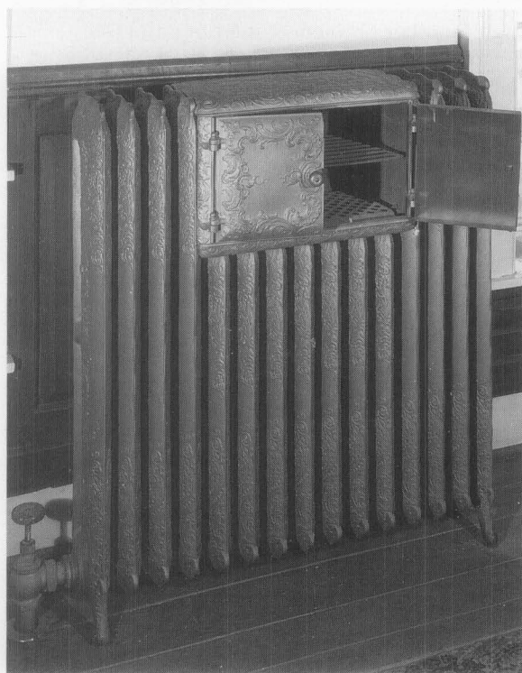
Figure 20. Historic metal components, such as this decorative cast-iron radiator, should be preserved during interior work. Following surface preparation, repainting with rust-inhibiting primer and finish coats is recommended. Photo: Jack E. Boucher for HABS.
