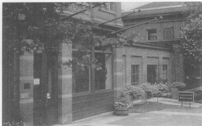
Figure 23. New additions to historic buildings can be designed to increase accessibility. A new addition links two adjacent buildings used for the Albany, New York, Visitor’s Center, and incorporates an accessible entrance, restrooms, and signage. Photo: Clare Adams.
