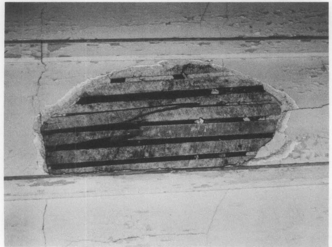
Fig. 13. This beaded ceiling in one of the bedrooms of the 1847 Lockwood House, Harpers Ferry, West Virginia, is missing portions of plaster due to broken keys. This is attributable, in part, to deterioration of the wood lath. Photo: Kaye Ellen Simonson.
