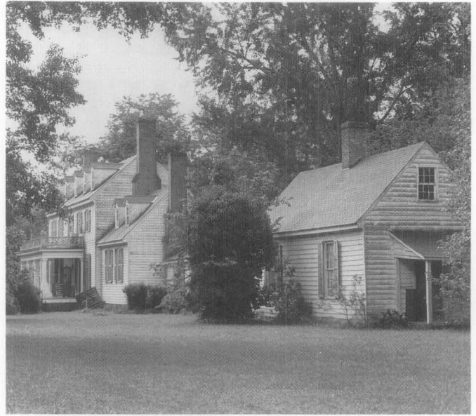
1. Eighteenth century and later vernacular architecture depended on the siting of the building, deciduous trees, cross ventilation, and the placement of windows and chimneys to maximize winter heating and natural summer cooling. Regional details, as seen in this Virginia house, include external chimneys and a separate summer kitchen to reduce fire risk and isolate heat in the summer. Photo: NPS Files.
