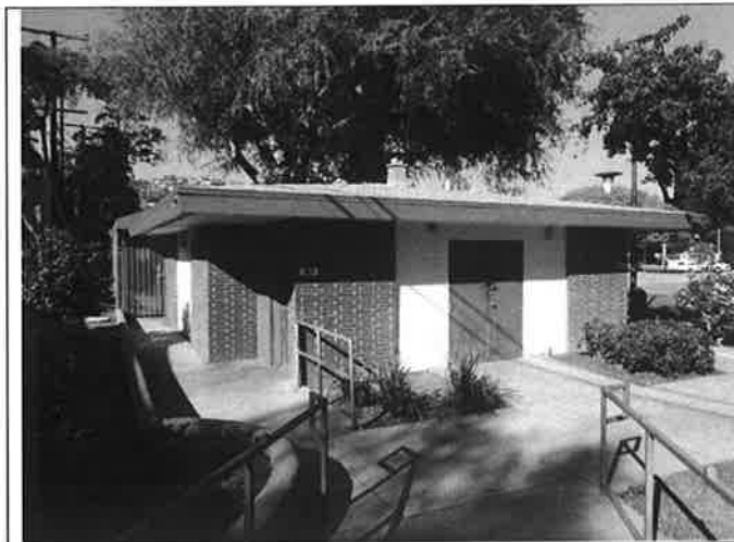
11. View of the public restroom structure
