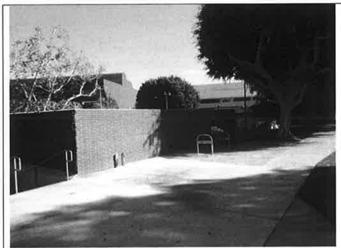
17. View of West Hollywood Aquatic Facility to the east
