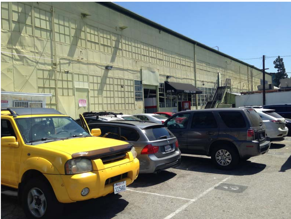
View of the subject property nightclub (2 nd floor) and gym (1 st floor) 650 N La Peer Dr, West Hollywood
