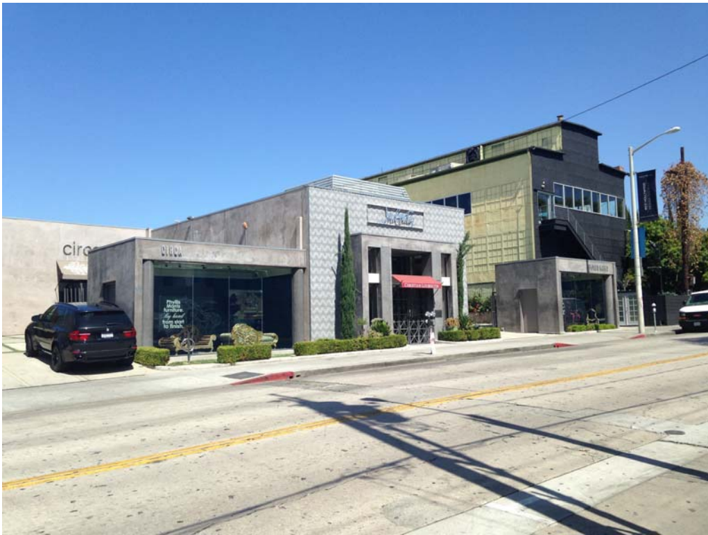
View of the subject property from Robertson Blvd (looking NW) 655-657 Robertson Blvd, West Hollywood
