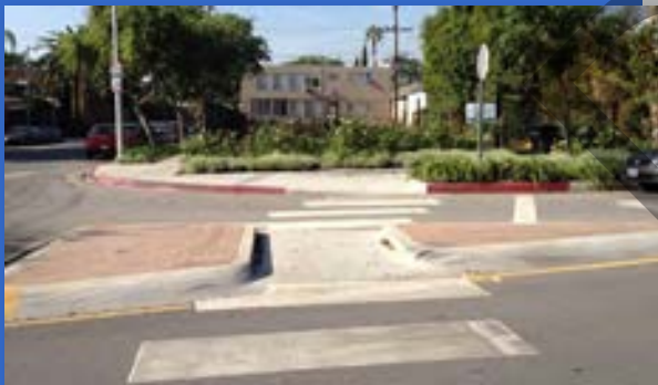
Pictured: Landscaped neighborhood traffic circle (top), Curb extension at Norwich Dr. (middle), A splitter island preceding a landscaped traffic circle at Detroit St. & Lexington Ave. doubles as a pedestrian refuge (bottom)
