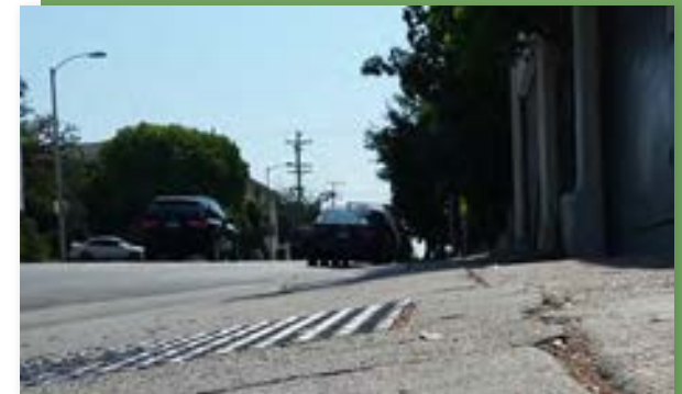
Pictured: Overgrown bushes narrow the pedestrian space and sight-lines around the corner (top & middle), sidewalk conditions are often sloping and uneven (bottom).
