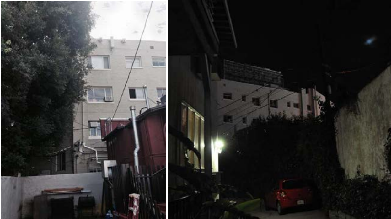
Figure 20: View of the Project Site from 1477 Havenhurst
