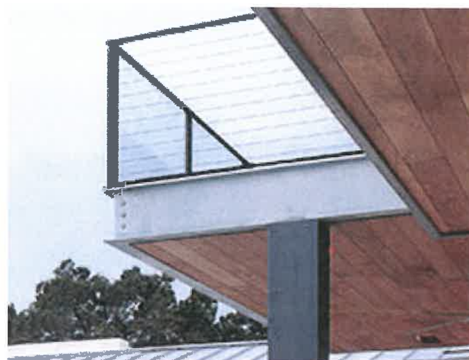
STEEL CABLE GUARDRAIL
