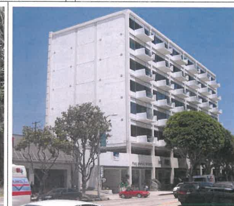
2 VIEW ACROSS BEVERLY LOOKING NORTH-EAST
