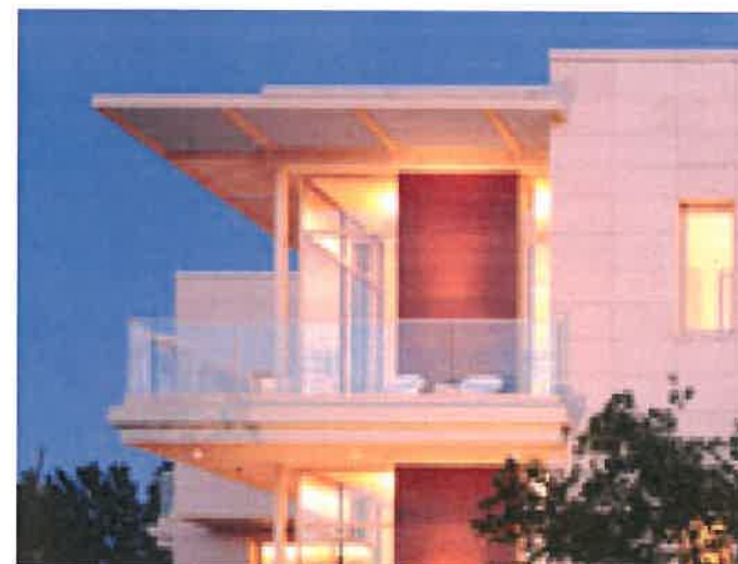
PAINTED STEEL OVERHANG
