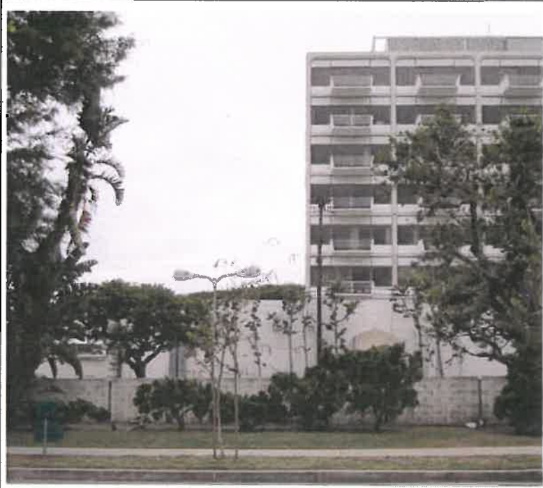
4 VIEW FROM ACROSS ROSEWOOD AVE. LOOKING SOUTH
