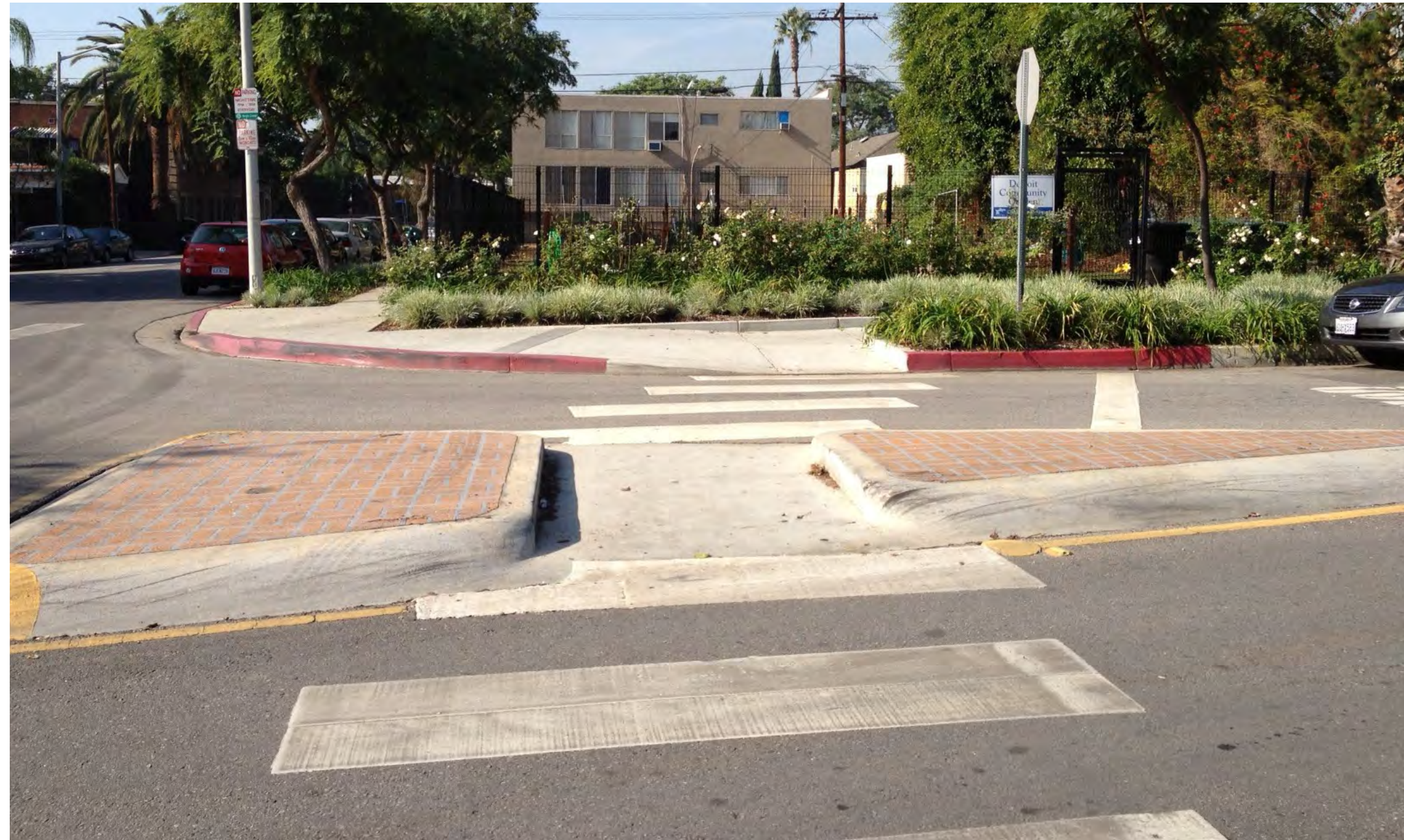
Pedestrian Refuge and Traffic Diverter, Detroit St. & Lexington Ave.
