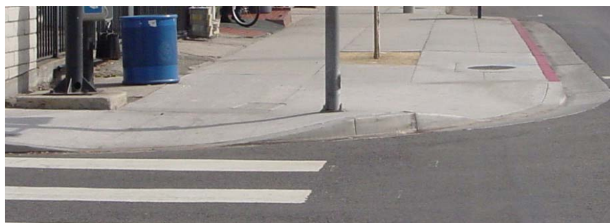
Figure 7.16 Dual Wheelchair Ramps
