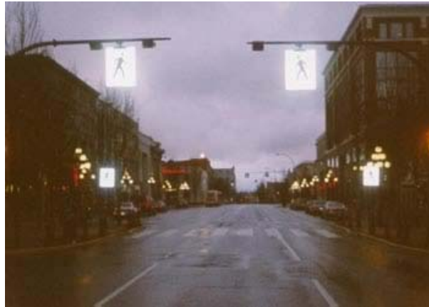
Figure 7.3 Example of an Overhead Crosswalk Lighting System
