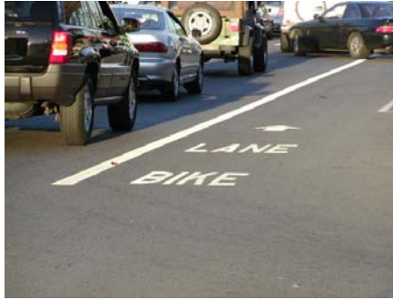
Figure 4.2 Class II Bike Lane Striping and Stencil
