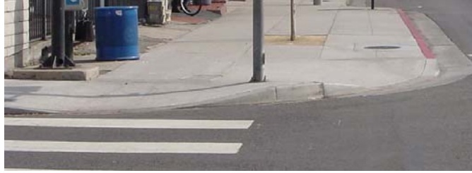
Figure 5.4 ADA-Compliant Wheelchair Ramp Design
